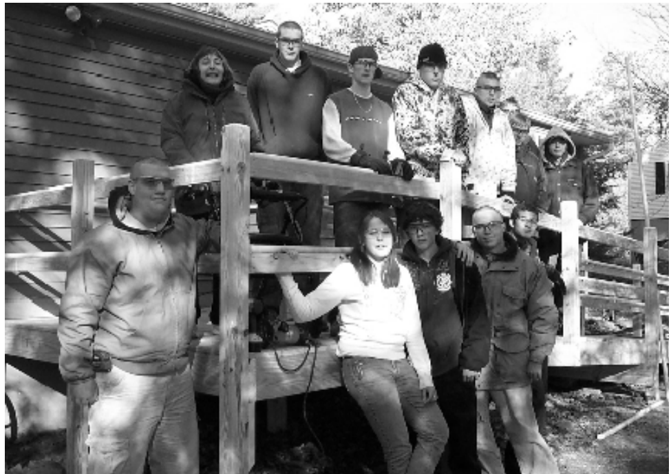
Mischelle Lach (upper left) poses with some of the Bay Path carpentry students upon the completion of her ramp.
